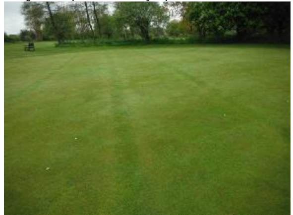
Figure 4: Surface levels along the tops of the drainage lines on the 13 th green had yet to be perfected
