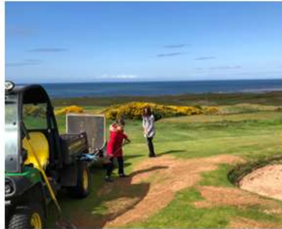
Filling in the dried out cracks on the newly turfed areas. With lockdown help
