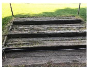
reconstruct each section of steps and replace with new sleepers or to apply non slip material to the existing steps it was agreed during an on site meeting that non slip strips should be applied to the existing steps. Costings have been carried out and once approved by Fusion Head Office this work will be completed to bring the steps back into play and to reduce risk of slips and falls in wet conditions.
