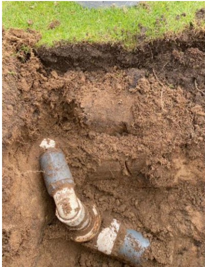
Digging up damaged pipes
