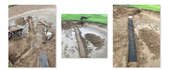
You will see the drain that has been put in needs to be maintained. It did not have a filter in it to allow water to drain away with the mud / silt etc. The black plastic is also acting as a filter and, as you can see by the photos it needs cleaning.
