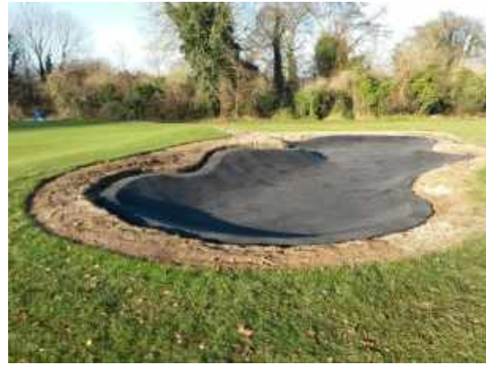
Figure 19 The liner complete ready for turfing the surround
