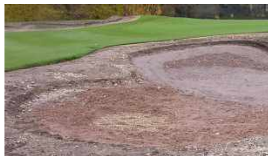
Figure 17 The foundation layers of the bunkers
