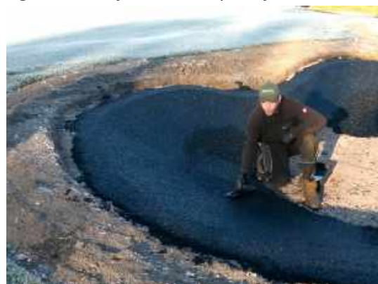
Figure 18 Laying the bunker blinder
