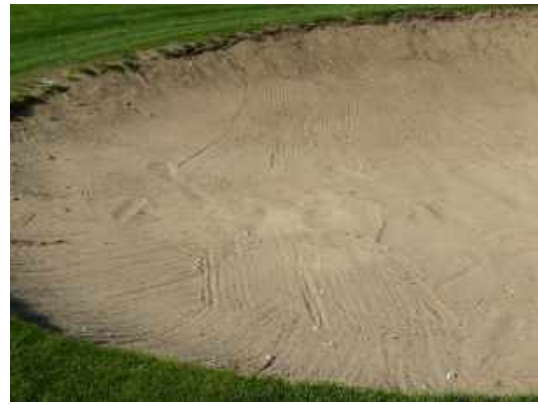
Figure 15 Chalk stones inevitably contaminate unlined bunkers from below
