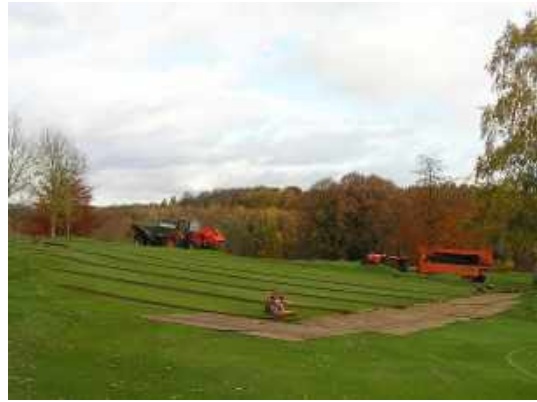
Figure 22 Removing the turf strips for the new drainage
