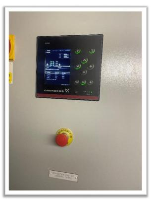
The newly replaced pump control panel is now fully operational.
