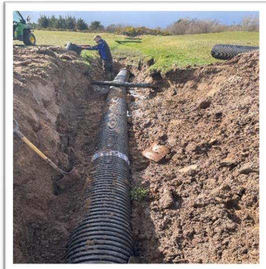
Pictures show where the irrigation pipe crosses the line of the pipe and the new pipe that was installed to replace the old clay pipe. As we had to dig the pipeline to the open ditch there was quite a bit of re-turfing required in this area. 160mts of turf was laid from our nursery to improve all worn turf in this area.
