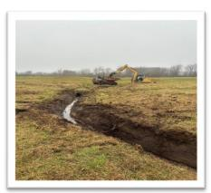
Clearance, redefining of the hazard edges and removal of debris in the burns/ditches at holes 5, 7, 12 and 14. (Pictured above in the middle & right-hand side)
