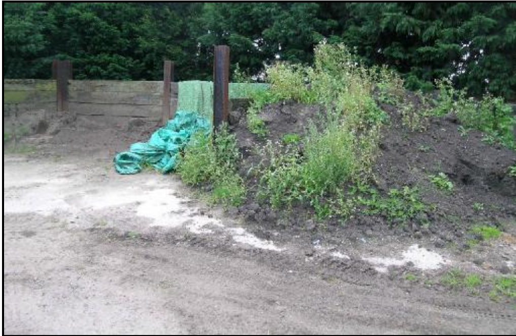
Figure 16: Additional storage bays are needed.
