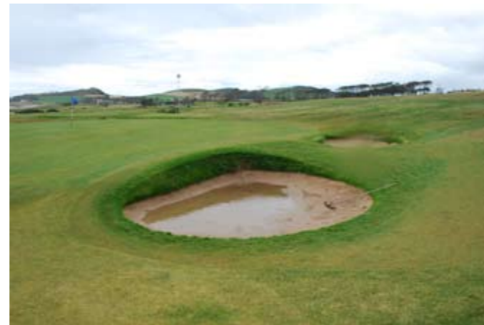
New bunker construction with drainage issues.
