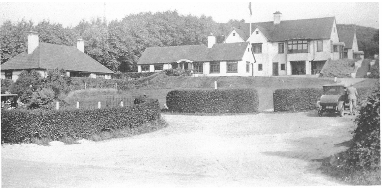
The steward's bungalow (left) was built in 1922. Between it and the clubhouse is the building which contained the secretary's office and ladies' changing room.
