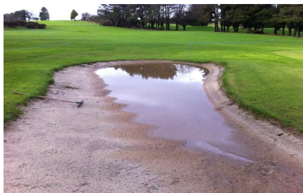
Ponding in Bunker - drain
