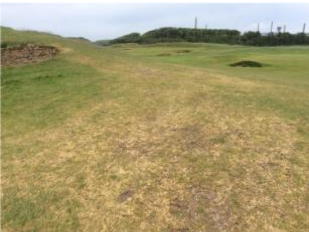
Figure 9: Dry soils and heavy compaction has resulted in a loss of grass cover to a number of sections of fairway.
