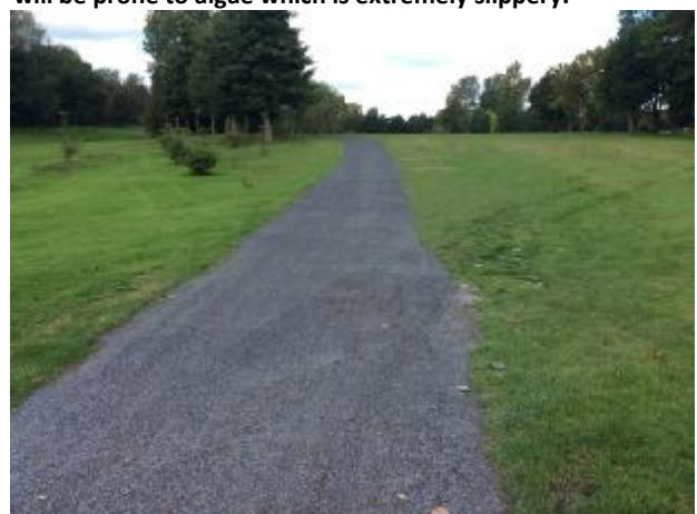
Figure 6: The Club have most sensibly invested in extending the grey shale path network. Some additional areas are to be included in this winter's programme. Ensuring access through periods of wet weather is critical.
