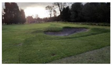
6th right-hand bunker. We have lowered the entrance off the bunker to make it easier to accesses in and out. We have also installed additional gull pots and a small swell to try and catch surface water from flooding the bunker.
